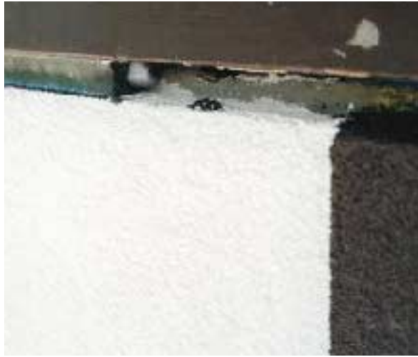
Figure 4. In a correctly executed butt joint — like the one in progress here — the edge of the insulation board is held back 1/2 to 3/4 inch, then backwrapped with mesh and base-coated. Note the backer rod and the well-tooled bead of caulk.
