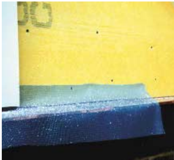
Figure 5. Headers and other horizontal surfaces must be protected with flashing. In this case, the damaged EIFS system has been stripped off, and a waterproof fiberglass-faced gypsum board screwed to the studs. The EPS board is attached to the sheathing with adhesive. Once the reinforcing mesh has been turned up at the front, the bottom edge of the sheet will receive a layer of basecoat.
